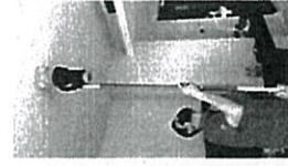
FL8 ROOM 803 TEST SMOKE DETECTOR 1 SET...NORMAL
