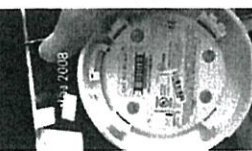
FL20 ROOM 2008 TEST SMOKE DETECTOR 1 SET...TROUBLE
